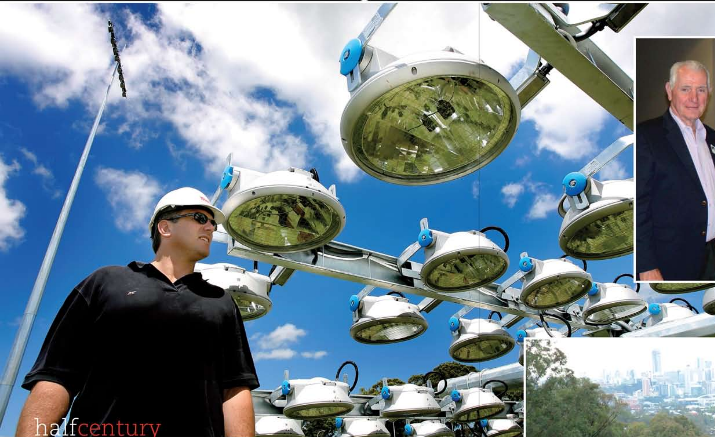
(1) 48 x 2000w Phillips arenavisions or 100,000 watts of lights on a 40 m pole at Corbould Park (image by Paul Smith) (2) Neil Fallon, Nathan Gundry & Mark Denning (3) Photoshoot at Mount Cool-tha with Brisbane in the background. Images supplied by Fallon Sevices and Paul Smith
